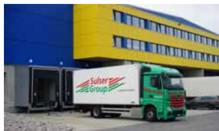
Sulser Logistics Solutions AG Logistikcenter Niederbipp Industriestrasse 3 CH-4704 Niederbipp / SO Telefon 0 844 40 20 40, info@sulsergroup.ch
